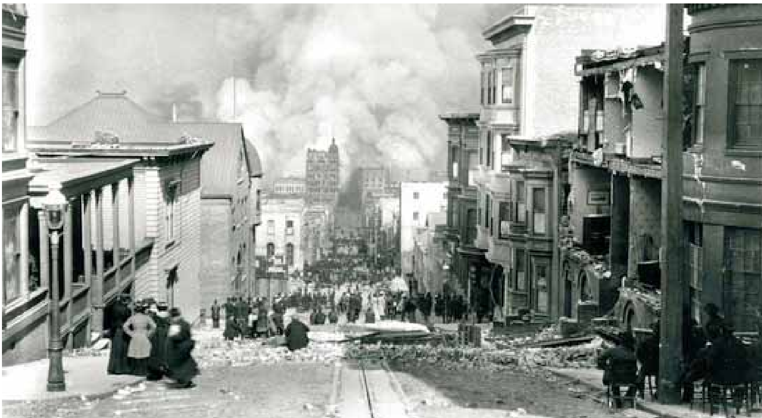
SCENE OF THE SAN FRANCISCO FIRE & EARTHQUAKE OF 1906
