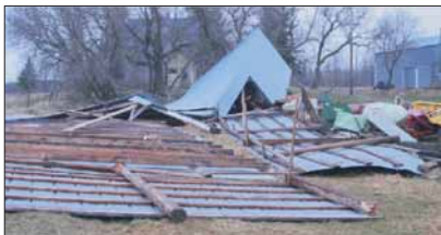
Dick Wilson's 25 year-old equipment shed.
