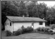
2799 Lost Lake Lane, on Lost Lake
