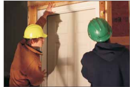
These men are making sure the door is set and flush
