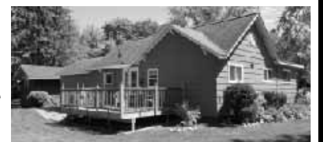
Rear view & new deck
