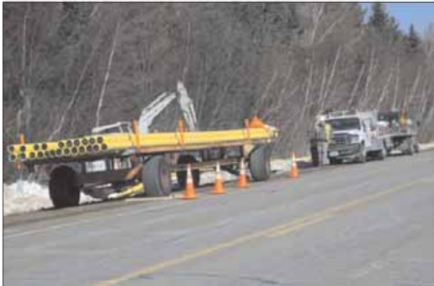
Crews at work on Hwy 32, north of Crandon
