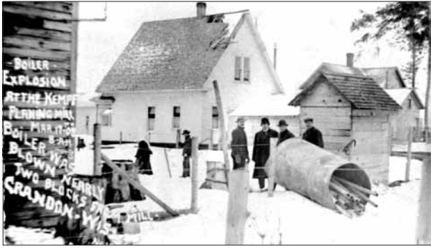
In the photo above, the boiler from the Kempf Planing Mill lays in the snow after bouncing off the roof of the house in the background. The date was March 17, 1908. It was the last day of operation for the mill, as the owner, Kempf, was killed in the explosion. Two more men were killed, and a third injured. This home still stands at 605 N. Hazeldell.
