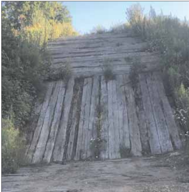
There could be slivers waiting for the runners on this nearly vertical climb made from ties.
