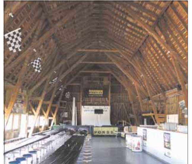
The original barn, located at what was known as "Plumber's Farm," was one of two structures on the property before becoming the legendary Crandon International Raceway (top). Much of the remodeling work will come to the building's main floor, including a new BFGoodrich heritage display, resurfaced walls and service bar, as well as the installation of numerous video monitors and an enhanced audio system (above).
