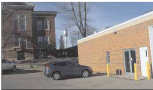
Prisoners that are taken to court leave by this door on right to the courthouse door on left. Dennee says that this can be a risk in today's society, not to mention a liability question in winter
