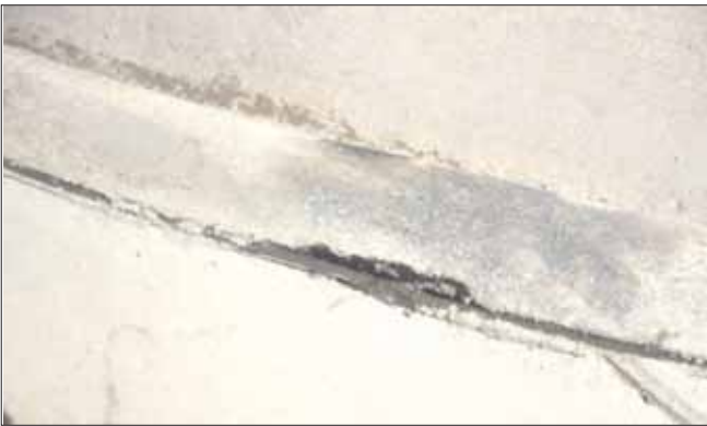
The matchup between the new curb and the sidewalk has a few flaws. On a simple walk around town, it is obvious that not much effort was made to give the city a nice, smooth sidewalk.
