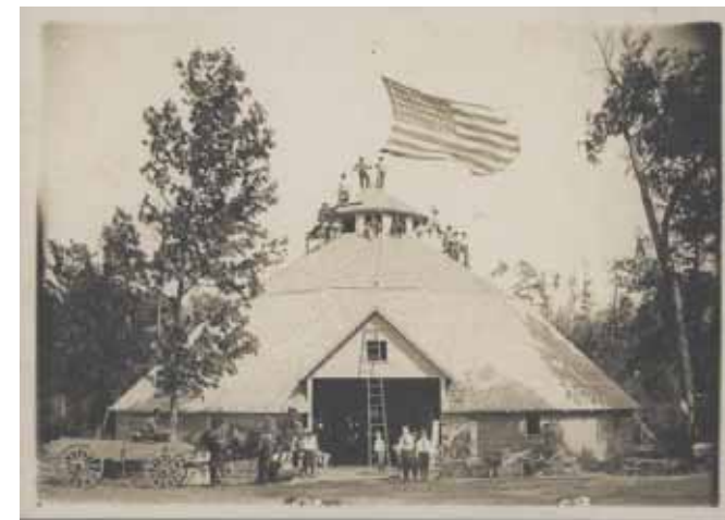
The original Forest County Fair barn that was torn down to build a new cattle barn in 1935
