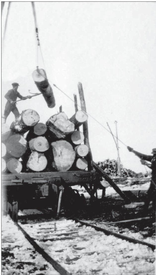
These guys are loading logs in Newald in the 1920's. If they were still around when hydraulic loaders came around, they would be amazed. One guy would do what three could do back in the a-frame loading days. It looks like this is actually a crew of four. There would be two more guys hooking up the logs on the left side of the car.
