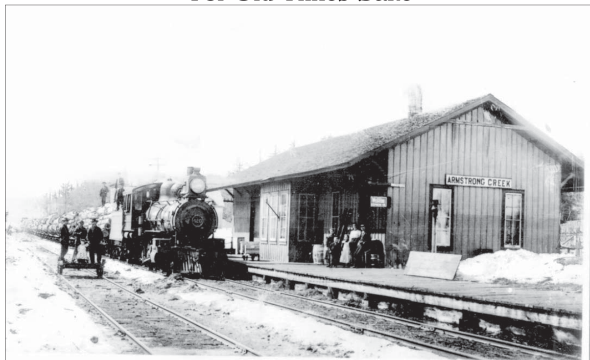
This was the hub of Armstrong Creek at one time. If you were going anywhere or just arriving, this is the first building you entered in Armstrong Creek. The Soo Line put Armstrong Creek on the map in 1887, along with Argonne and all the other towns along the new rail line. It was the door to the outside world. There was no Hwy 8, and nobody had a car anyway. This railroad and depot was actually the gateway to the rest of the world. As can be seen, the train is loaded with logs headed to the sawmill. And, if you wanted to take in a Broadway play in New York, the train is how you got there. This likely didn't happen too often.
