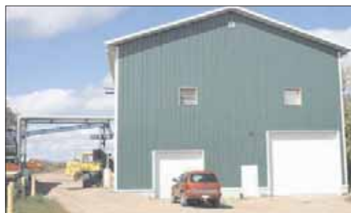
This new building houses the new boiler system. Pipes on left carry steam to the dry kilns.
