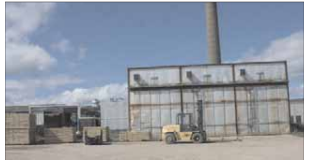
Three of the five kilns heated with the new boiler. The old landmark smokestack behind the kiln won't be smoking anymore.
