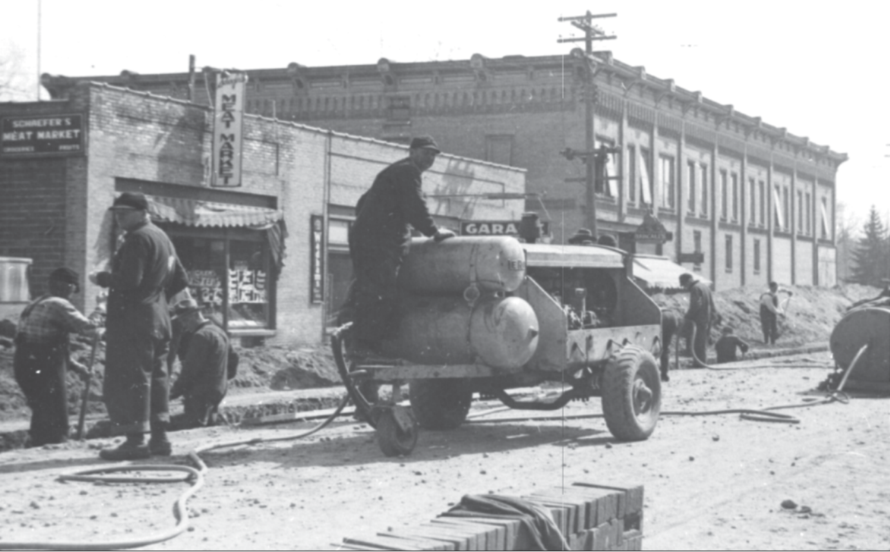
Crandon's main street seems to get more than its share of construction in recent times, but it went through it back in the 30's as well. We think this is when water and sewer was installed. Notice that Freimuth's garage shows up as does Schaefer's Meat Market. If someone would combine those two buildings, it would make a great bank. Wait! They did that in recent times. Those two buildings on the left are now the Laona State Bank. The big building that now houses Subway and other businesses, was a grocery and theater in those days.
